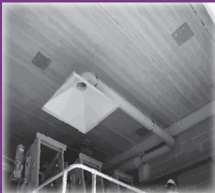
Bell gas extraction
