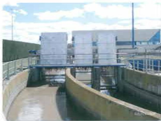
When intense rainfall causes the flow to increase to above the maximum rate capable of being dealt with by the processes, the excess water is sent to a stormwater tank with a capacity of 7,500 m<sup>3</sup> for the purpose of storing first flush rainwater, which has washed roofs and streets, so that this water can be treated subsequently when the inflow to the plant has decreased.
