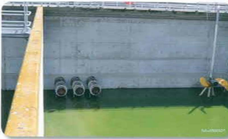
mm. This waste is deposited into containers for subsequent landfilling. Then, in four parallel channels, grease is removed through floatation by means of air bubbles injected into the lower part of each channel. The grit, which sediments to the bottom of these channels is also removed.
