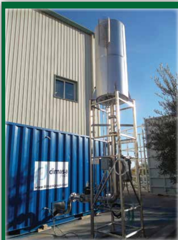
Biogas Combustion Plant, Exterior view
