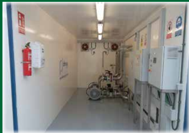
Biogas Combustion Plant, interior view
