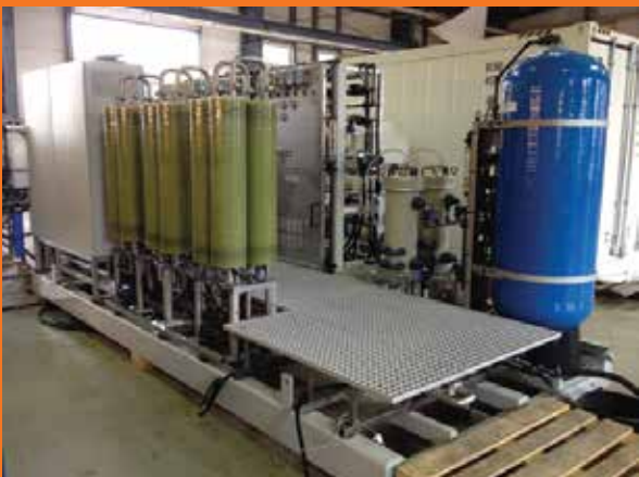
Leachate treatment plant
