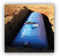
Compact SBR plant technology has based on the same principle as extended aeration TOP plants but in the same chamber it is performed the aeration and decantation in a sequence mode.
