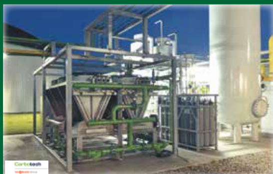
Biogas Upgrading Plants
